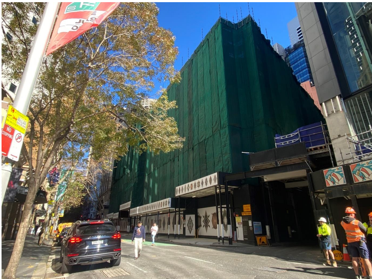
Figure 2: Existing site under demolition as viewed facing south along Pitt Street
